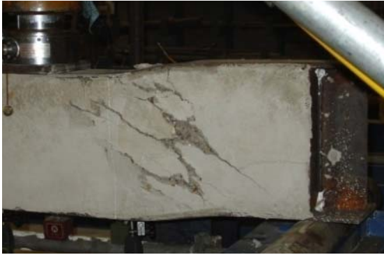
Figure 7. USFB No.1 at Failure point.
