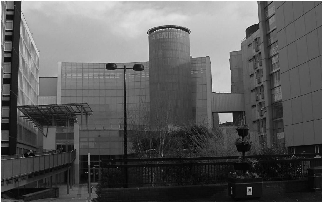
Figure 1. The Saltire Centre – Front Elevation
