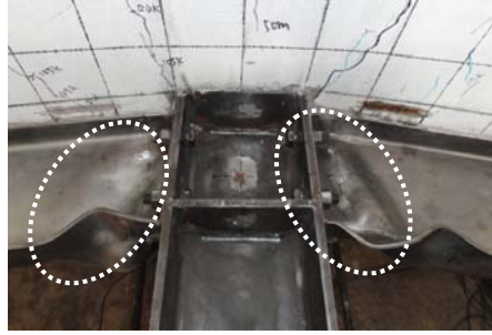
(b)Buckling of steel beam
