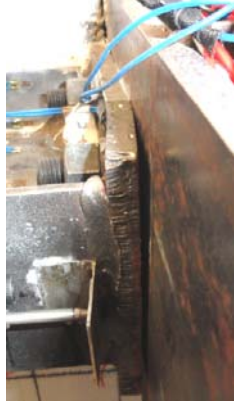
(a) Deformation of the endplate
