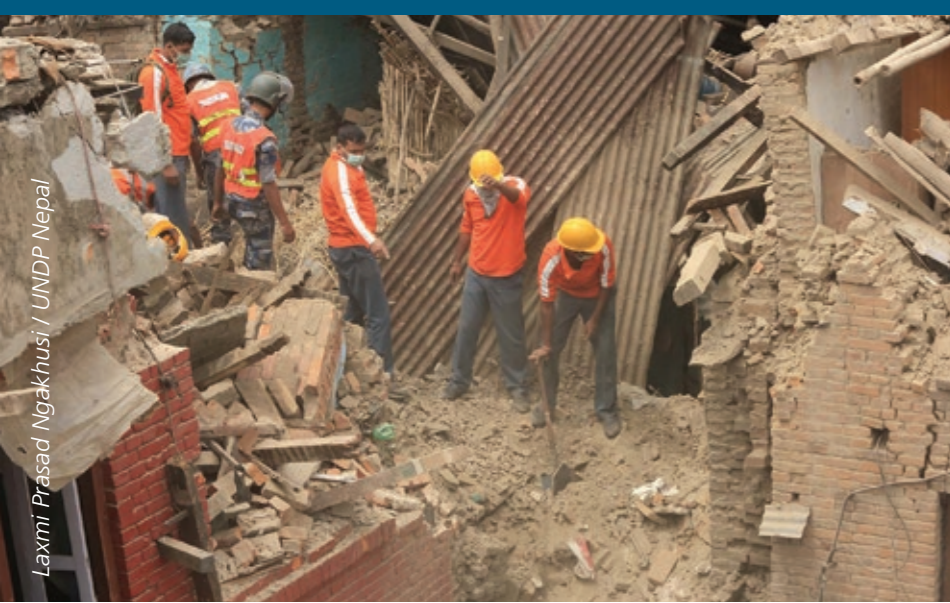
Some of the damage in Bhaktapur.
