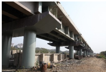
Figure 4. Mumbai railway viaduct
