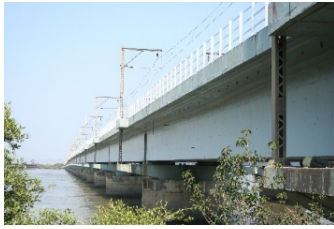
Figure 2. Mumbai railway bridge
