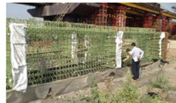
Figure 5. Sensors on reinforcement cage
