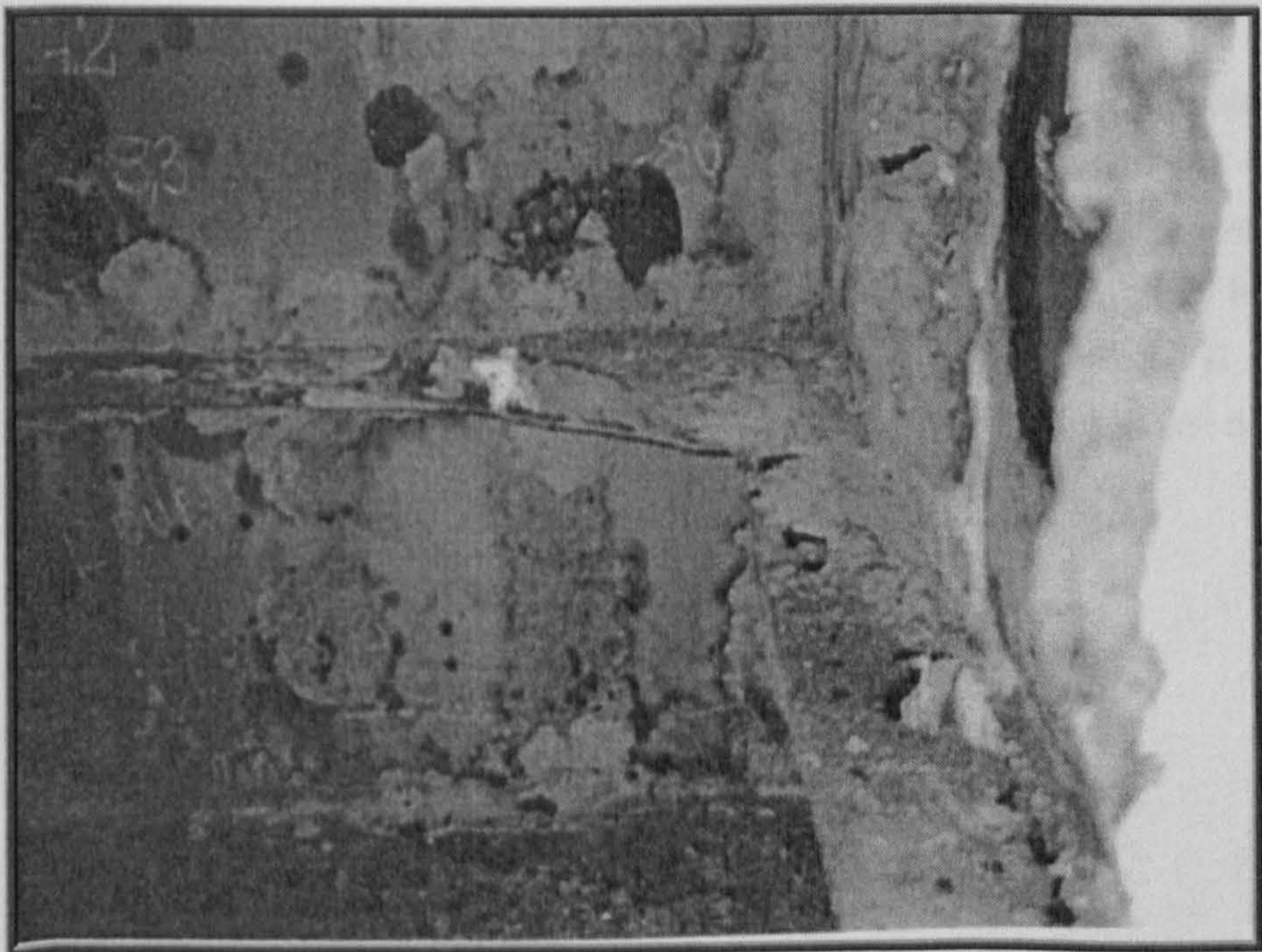
Figure 8-2 Combination of Fatigue Cracks and Localized Corrosion (Tanker Structure Co-operative Forum 1997)
