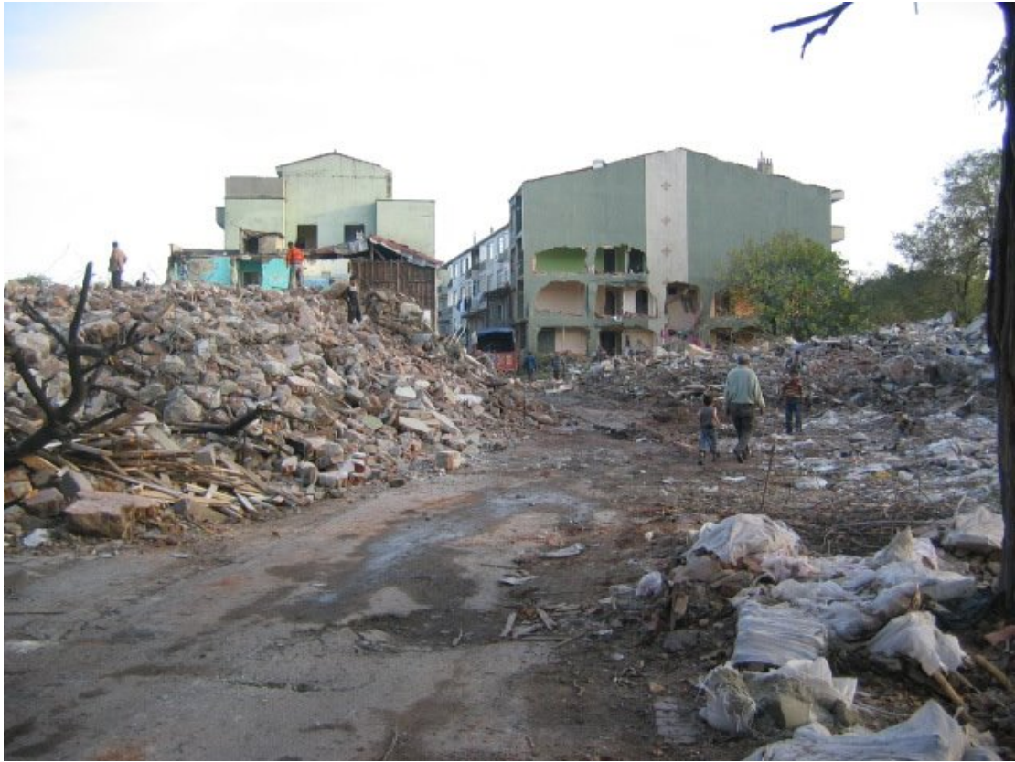
Fig. 14 – View from the demolitions of 2008. (Photo by: Özlem Ünsal)
