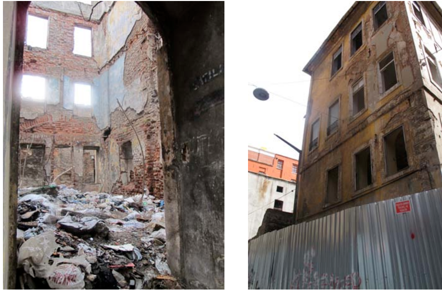
Figures 35 and 36 – Demolitions in Tarlabası, April 2013. (Photos by: Özlem Ünsal)
