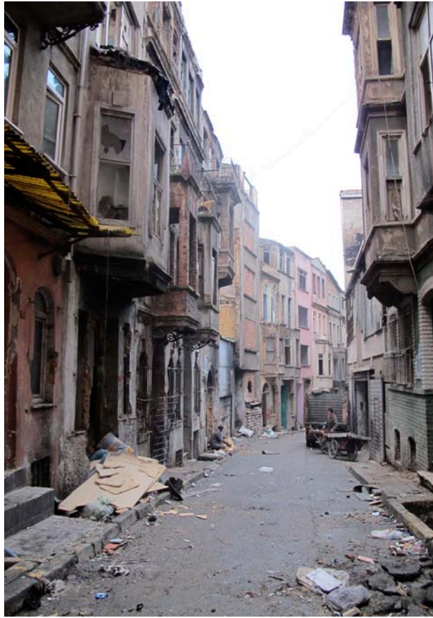
Fig. 40 – Image shows Tarlabası under demolition in February 2012 (Photo by: Özlem Ünsal).
