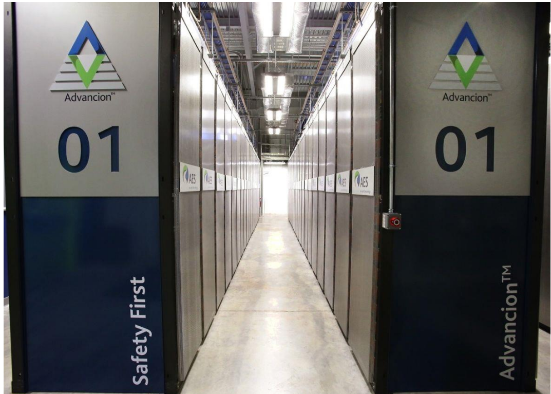
Figure 2.3. Grid-scale battery storage array in Kilroot, Ireland
