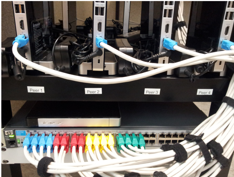
Figure 4.2: Photograph of the testbed with 32 peers, 1 controller peer, and a separate switch. Source: own representation.
