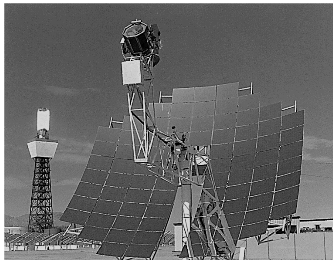
Figure 2.10 McDonnell Douglas (currently Boeing) Dish Concentrator; Daggett, California; USA (courtesy NREL). The Solar One Tower which is powered by a heliostat field is in the background.
