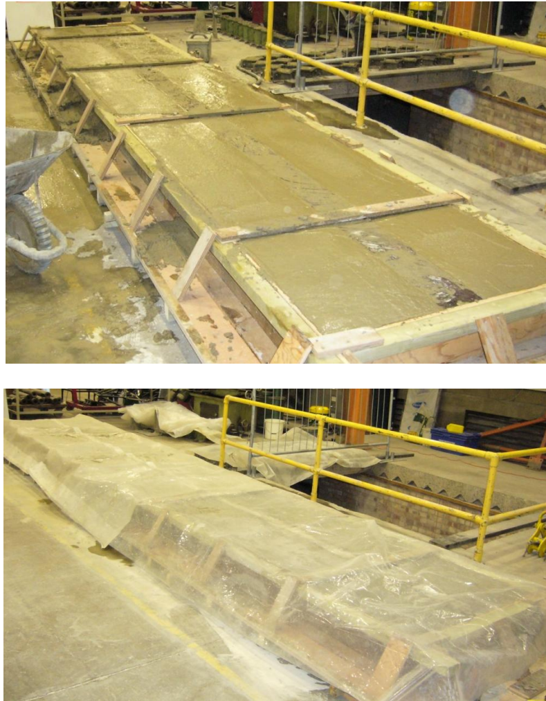
Figure 6.3 Casting and curing of the test beam specimen
