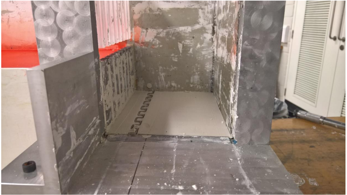
Figure 4.26 Photograph of double wall at formation level
