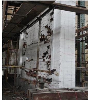
(b) back view of wall collapse
