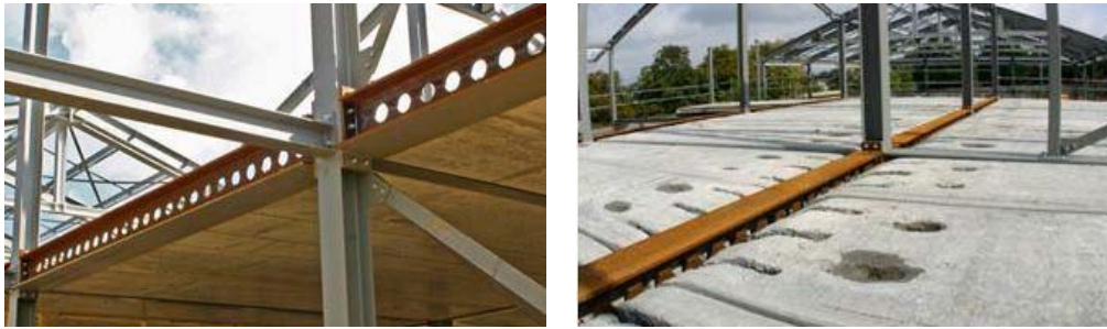
Fig. 2: USFB™ used with precast
