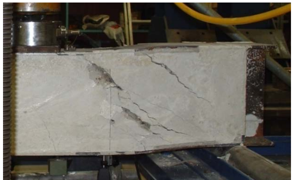
Figure 10. USFB No.4 at Failure point.
