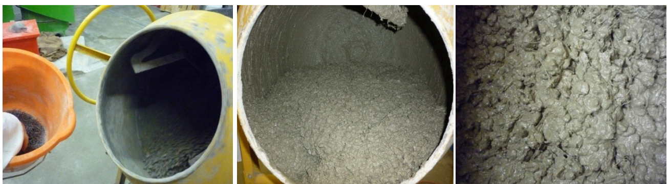
Figure 19. Adding steel fiber to the mix
