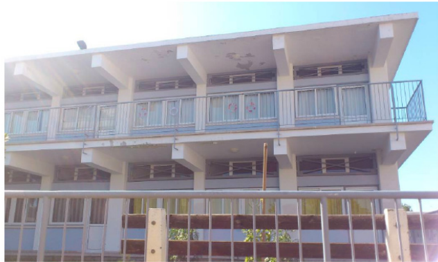
Fig. (15). Back view of the selected strengthened R/C building.
