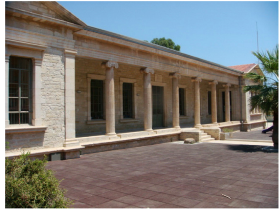
Fig. (17). Front view of the selected Masonry building.
