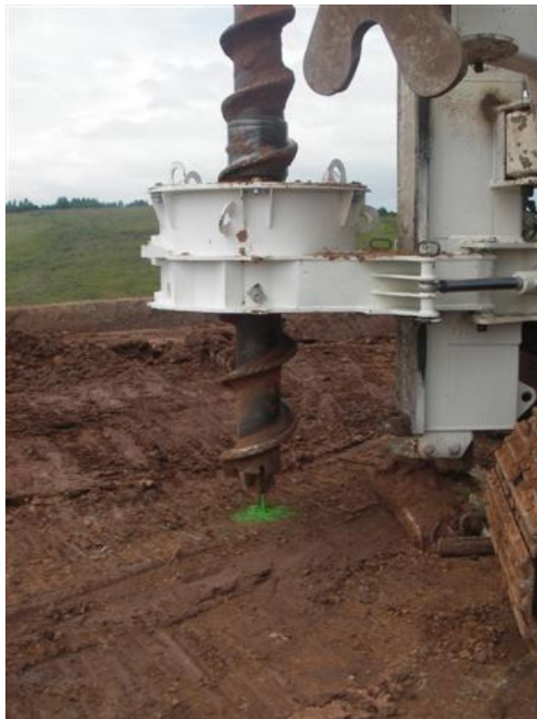
Figure 3.5 The auger used to install test piles
