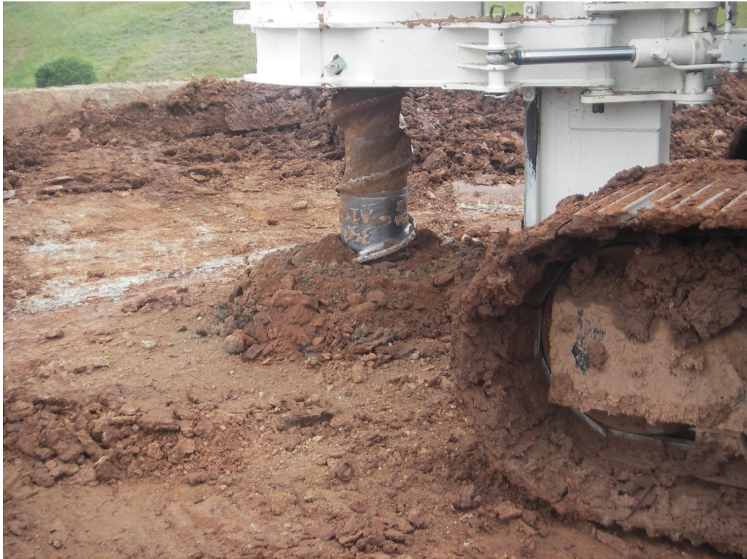
Figure 4.2 Risings during augering of pile MR1 and shows sharp angular blocks of hard material mixed with fine, red/brown powder, as seen while the auger was screwing into the soil
