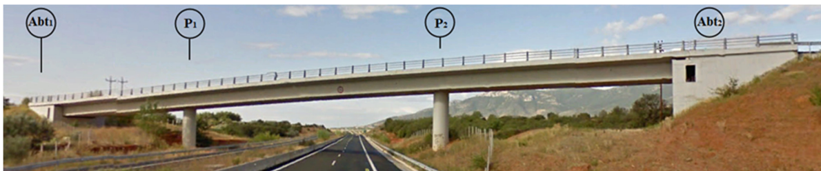
Figure 3: Studied bridge (Overpass T7, Egnatia Motorway, N. Greece)
