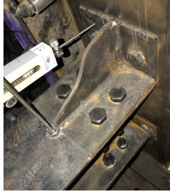
(b) Buckling of stiffener at top angle
