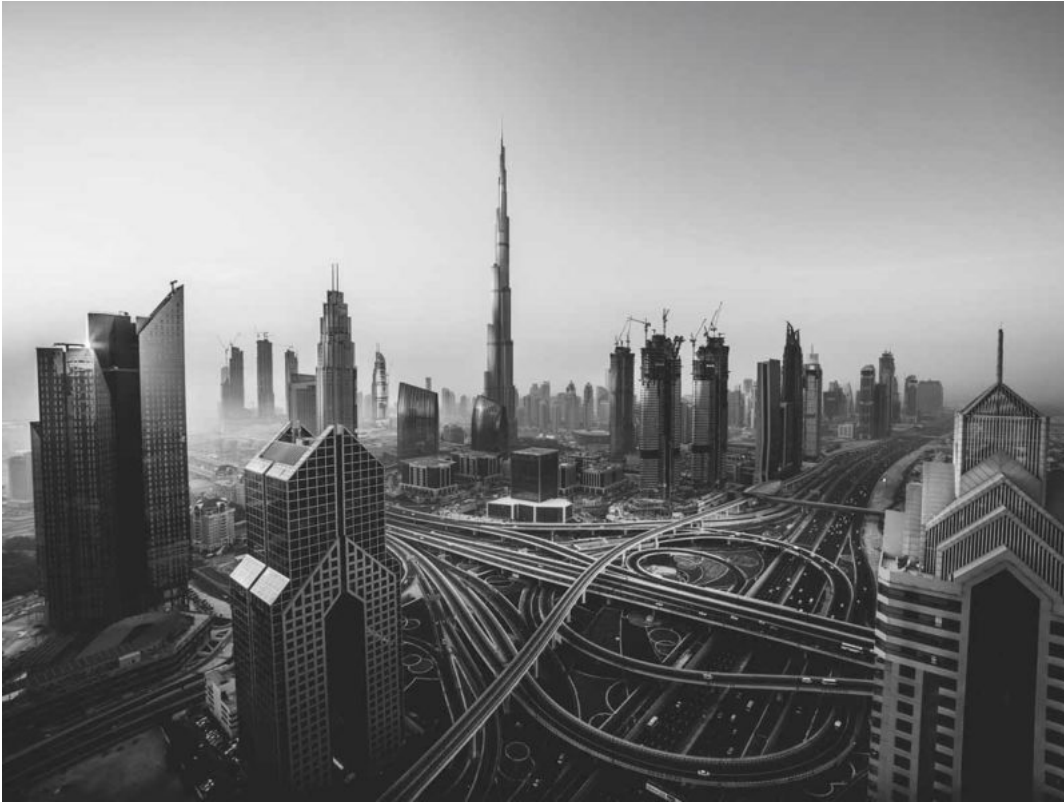
Figure 1.10: Buttressed core configuration of the Burj Khalifa (centre), Dubai
