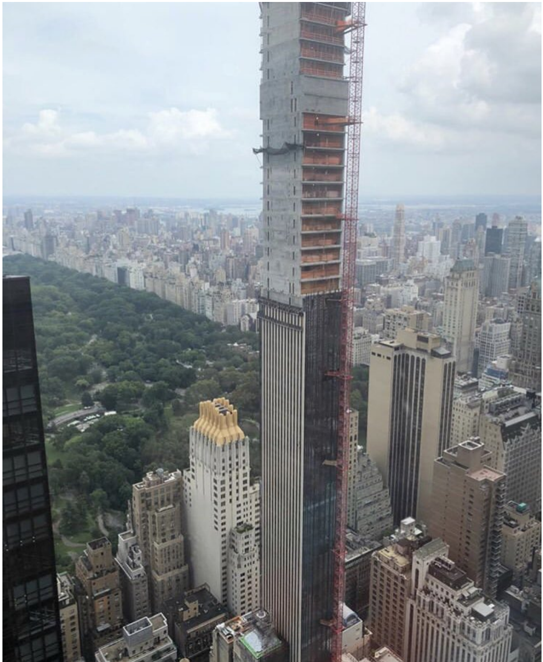
Figure 1.3: 111 West 57 th under construction
