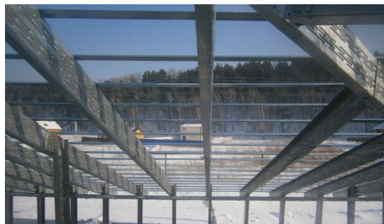
565 566 567 568 569 570 571 (a) Application of slotted perforated CFS channels
