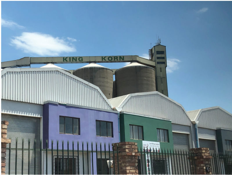
Figure 3. The towers of the King Korn processing plant of Tiger Brands in Potchefstroom (Source: Author's Own).
