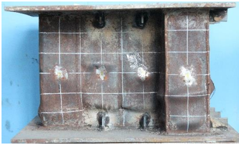
(c) Buckling mode of specimen CSW-T-1 (web)
