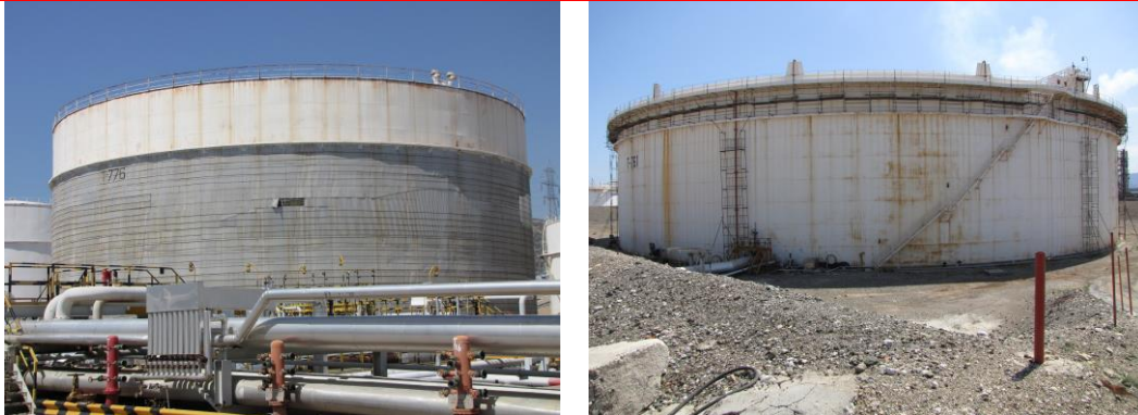
Fig. 1 On-site pictures of tank T-776 (left) and tank T-761 (right)
