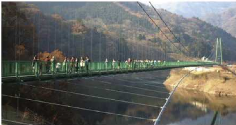
Fig. 6. View of the Nasu Shiobara footbridge in Japan (M-bridge)
