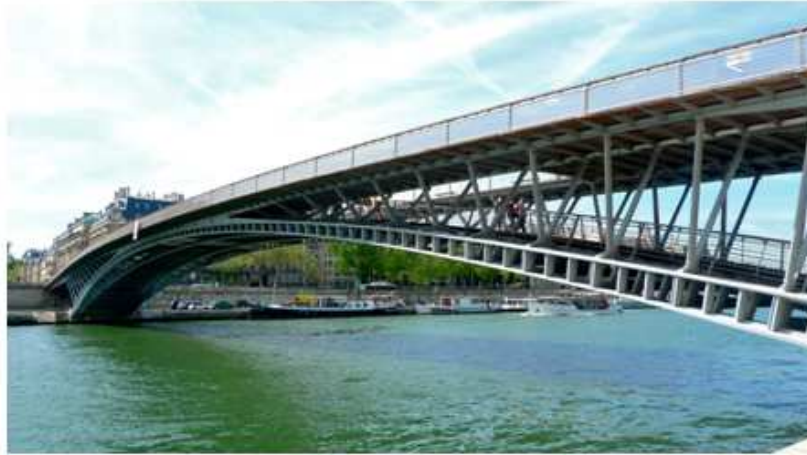
Fig. 5. View of the Solferino footbridge in Paris
