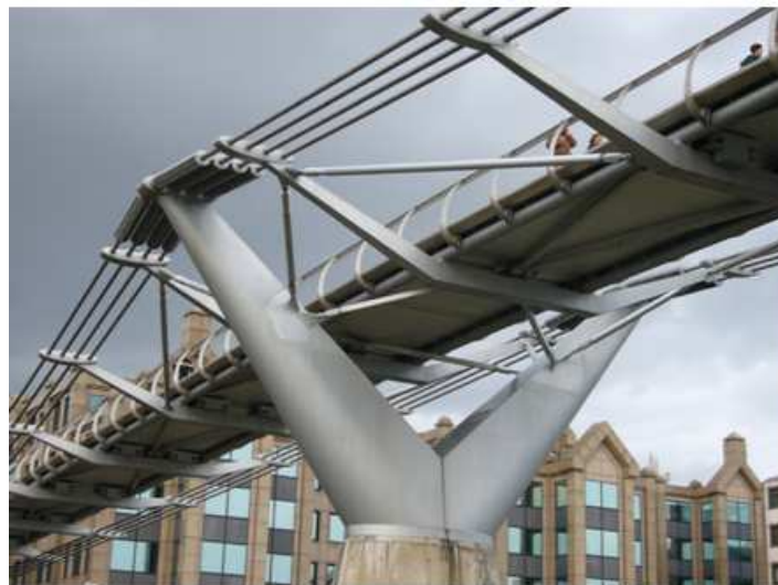
Fig. 4. View of the London Millennium Bridge (Brownjohn et al. , 2008)
