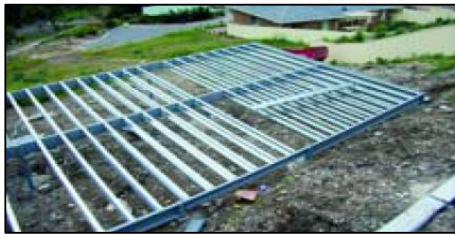
(a) Application of CFS as floor bearers
