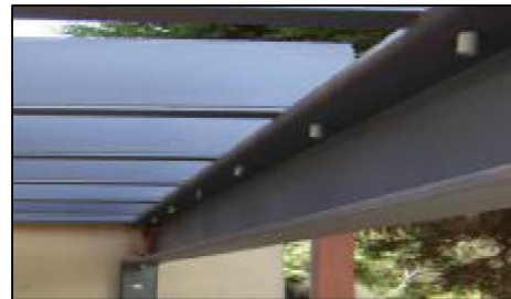
(d) Application of CFS as joists
