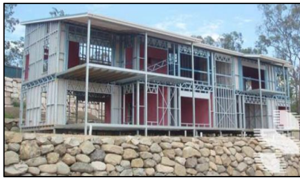
(c) Application of CFS as rafters
