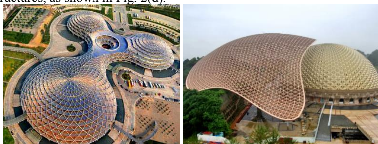
(a) Pearl Stadium, China
