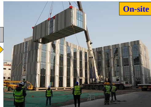
Hoisting of modules finished in six days
