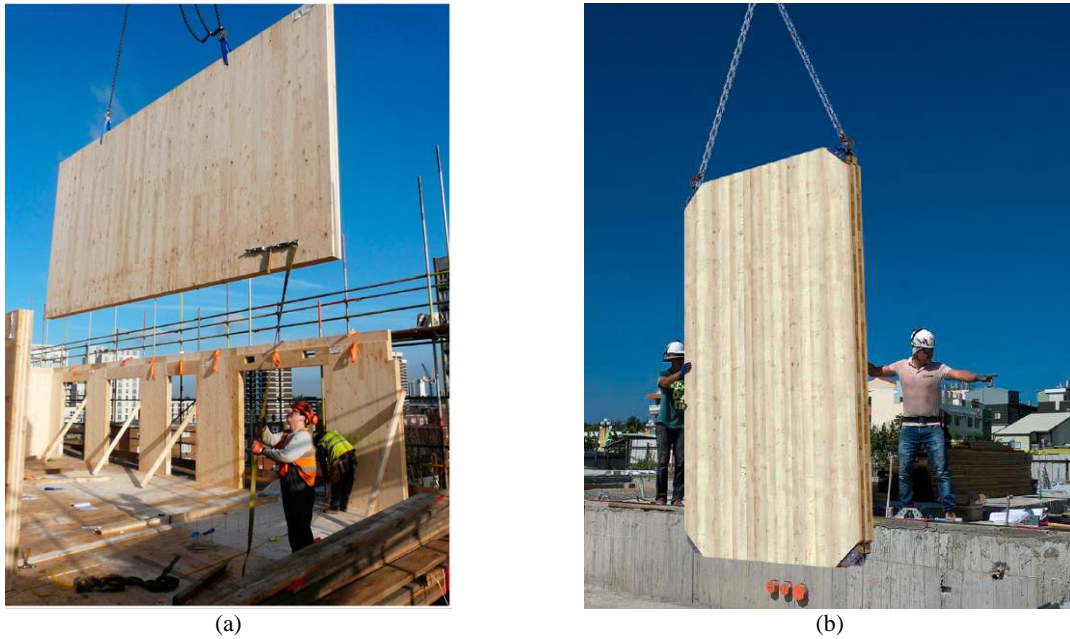
349 Figure 7. Panel lifting with (a) conventional method [86] and (b) novel connectors (CLT-C2) [60]
