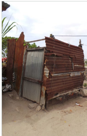
FIGURE 1 A pit latrine in Mji Mpya before the implementation of the Simplified Sewerage System
