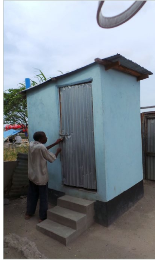
FIGURE 2 Improved toilet in Mji Mpya after the implementation of the Simplified Sewerage System
