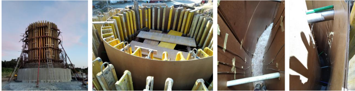
Figure 6.36: TT demo CAC formwork and FOS integration before pouring the CAC.
