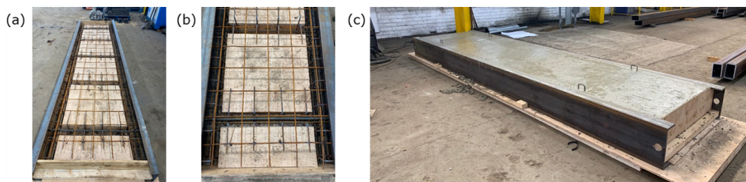
Fig. 3: (a), (b) Prepared Specimen before Casting Concrete (c) Casted Specimen
