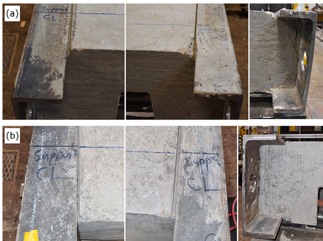
Fig. 21. Separation between steel and concrete at the end of the tests for (a) NWC-230-SD and (b) LWC-230-SD.
