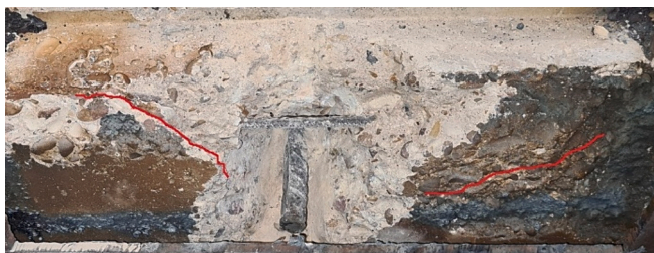
Fig. 19. Cracks in concrete near the failed shear connectors in NWC-300-SD.
