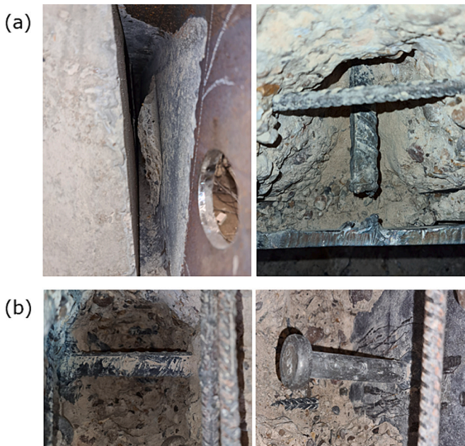
Fig. 18. Condition of (a) failed and (b) undamaged shear connectors after the test for NWC-300-SD.
