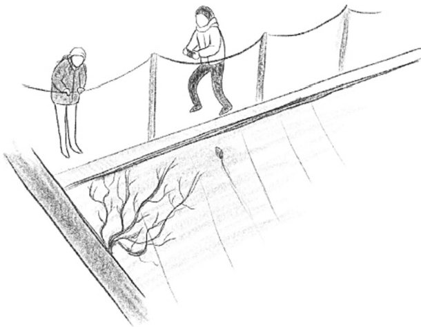
Fig. 7. “Then we sighted something very interesting: A tree growing from a crack in a vertical concrete wall!” (Fjeld et al., 2021: 5).
