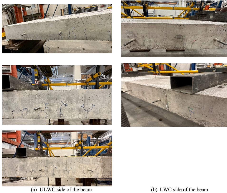
Fig. 11. Concrete crack development.
