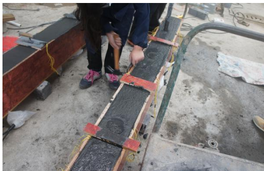
(c) Pressurization around timber forms
