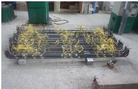
(a) Reinforcing cage
