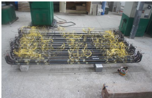
(a) Reinforcing cage
