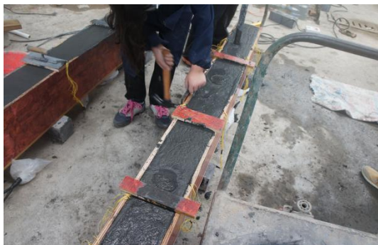
(c) Pressurization around timber forms
