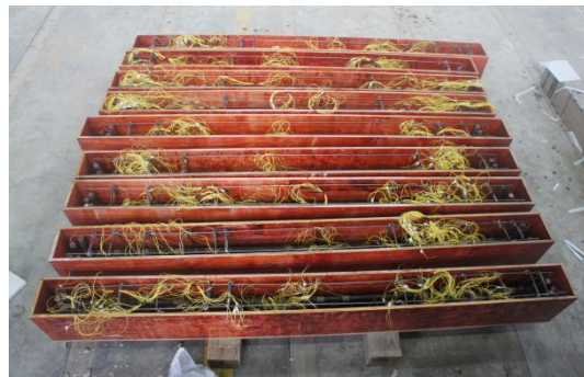
(b) timber forms
