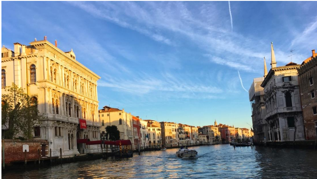
Figure 5.10 Palazzo Vendramin Calergi in Venice (left)
