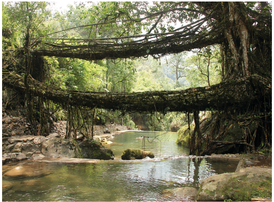
Living root bridge in Meghalaya, India. This design reframes the assumption that an organism needs to be killed before being utilized as a material in design. It remains unclear, however, how the principles of this design be scaled.
