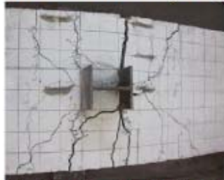
h) Crack on the slab of inside joint B
