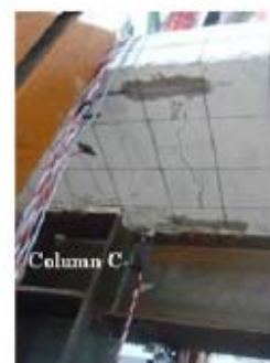
d) First crack around column C
