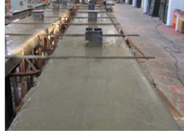
d) Concrete casting
