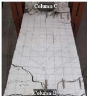
h) Diagonal cracks on the span of B-C
