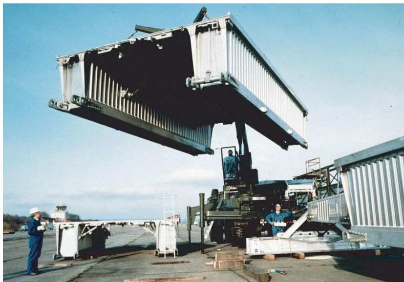
Figure 2: A German prefabricated aluminium military bridge during erection phase (Mazzolani, 2006).
