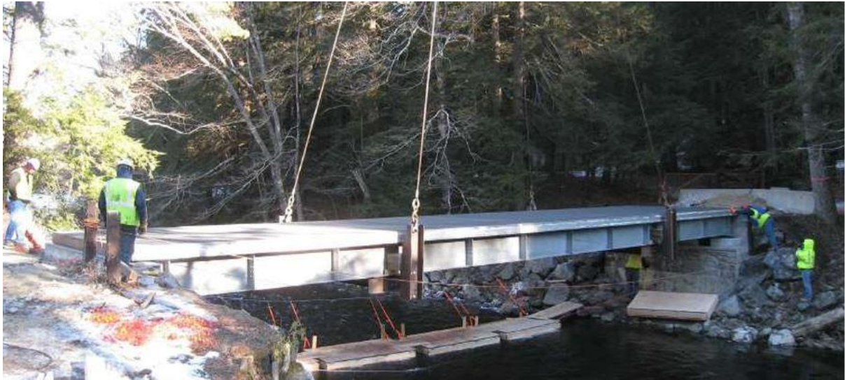
Figure 3: Sandisfield bridge (AlumaBridge, 2022).
