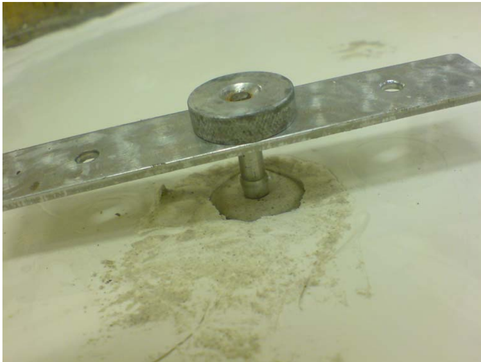
Figure 6.37 Photograph showing resin residue on clay surface around pile head
