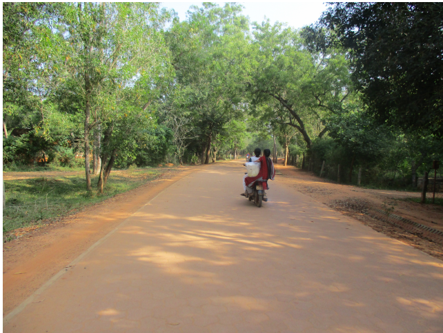
(b) Roads made with compacted earth or laterite soil with minimum asphalt coverage and rainwater drainage channels.
