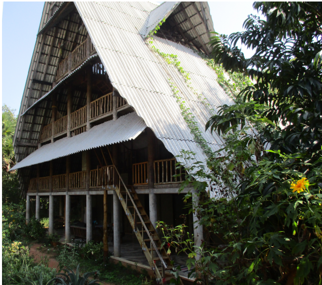
(b) Eco-friendly buildings built utilising local materials and earth construction techniques.
