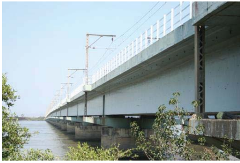
Fig. 4. General view of Vasai Creek Bridge.
