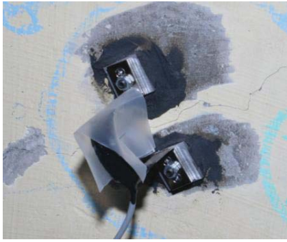
Fig. 9. Crack width sensor used in the bridge tests.
