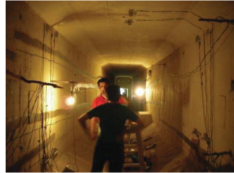
Fig. 6. View inside the box girder showing the scale and the environment in which the sensors are mounted.
