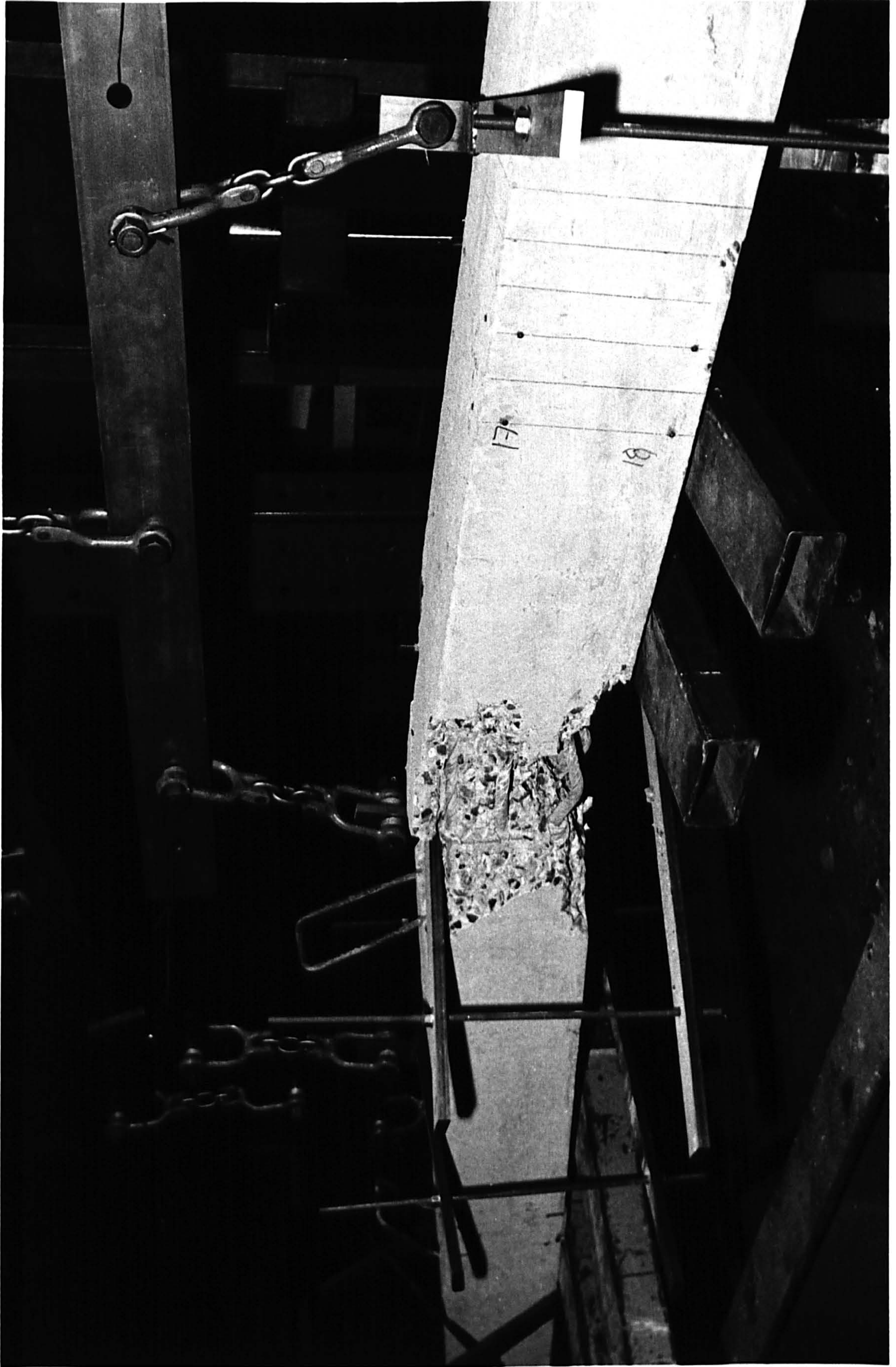
Fig. 4.7. View of the mode of failure
