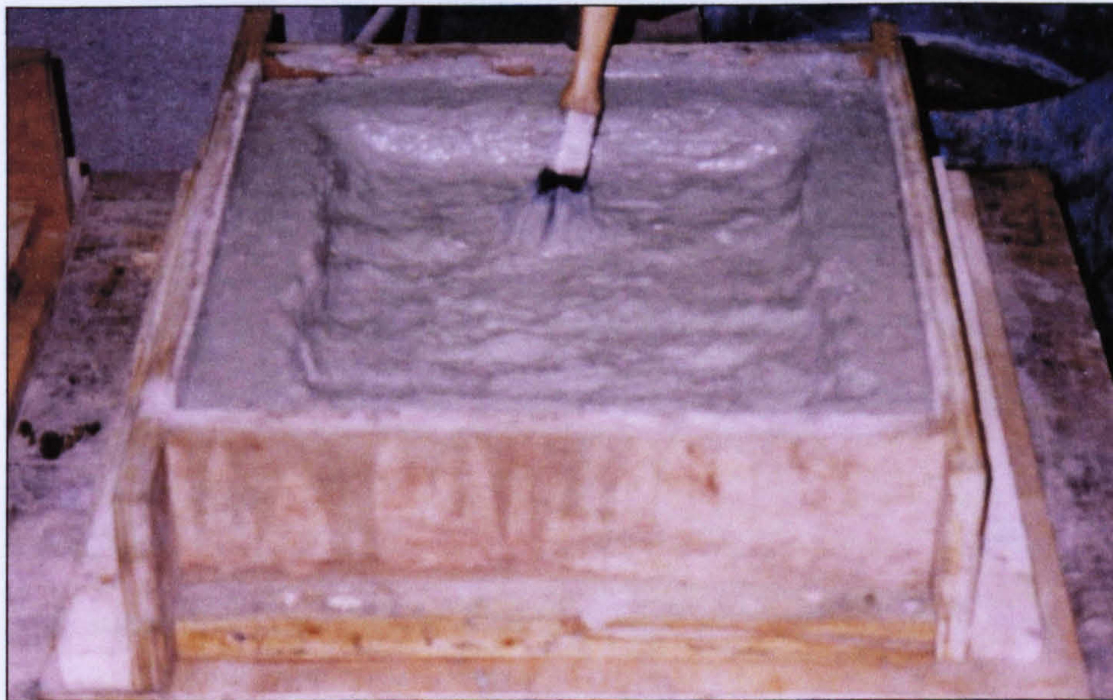
Application of bonding agent/primer Zentrifix KMH
