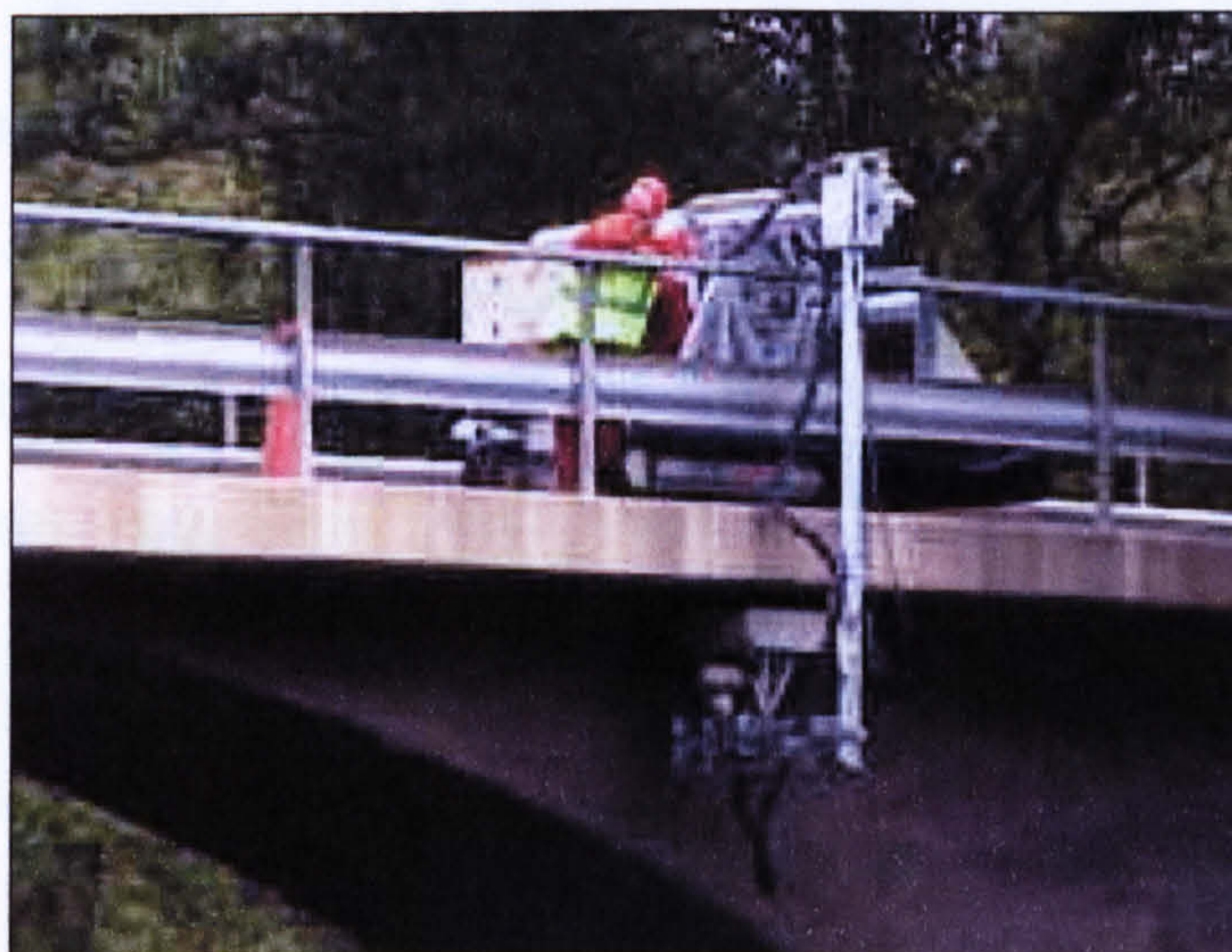
Figure 2.4 Hydrodemolition of a bridge pier in Sweden
