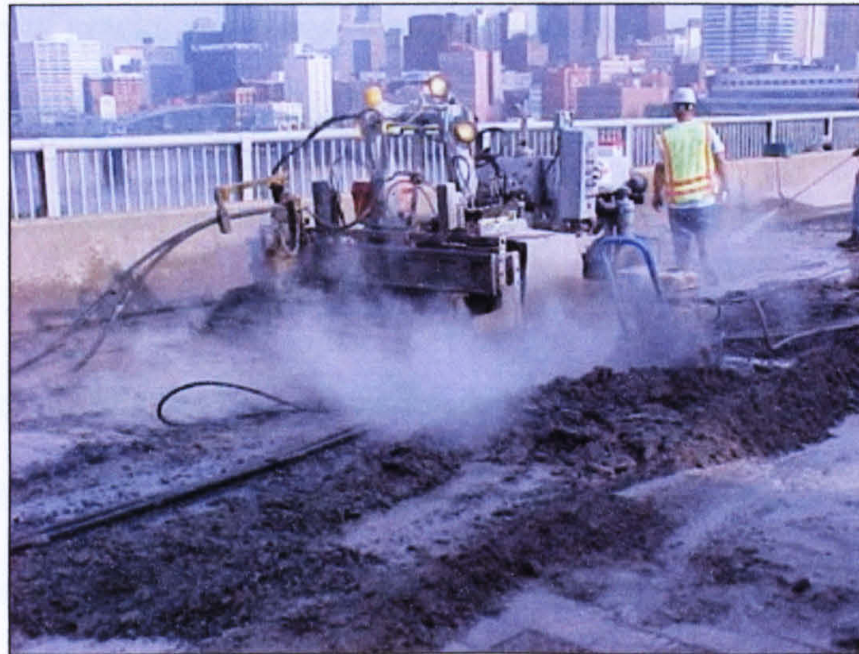
Figure 2.3 Removal of defective concrete from Liberty bridge in USA
