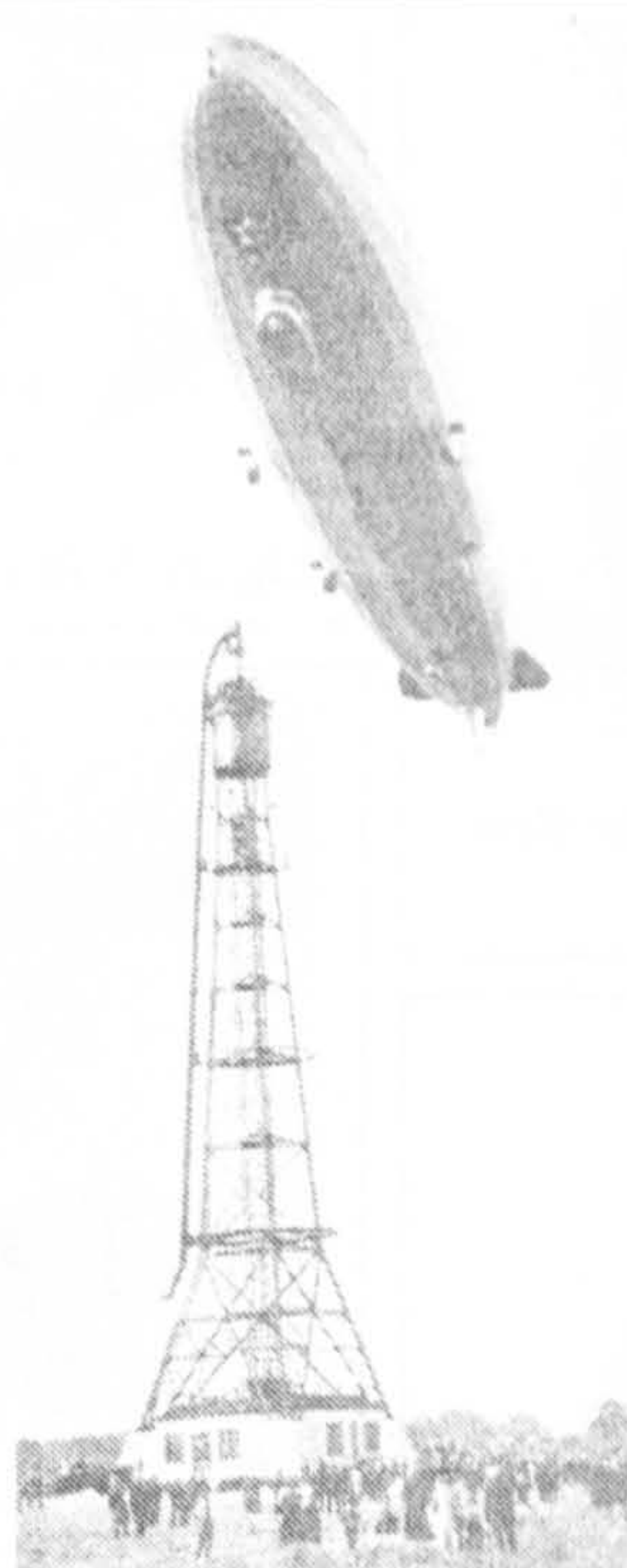
Figure 6.38 :1926 LZ126 at Ford’s Dearborn mast with “vertical railway”
