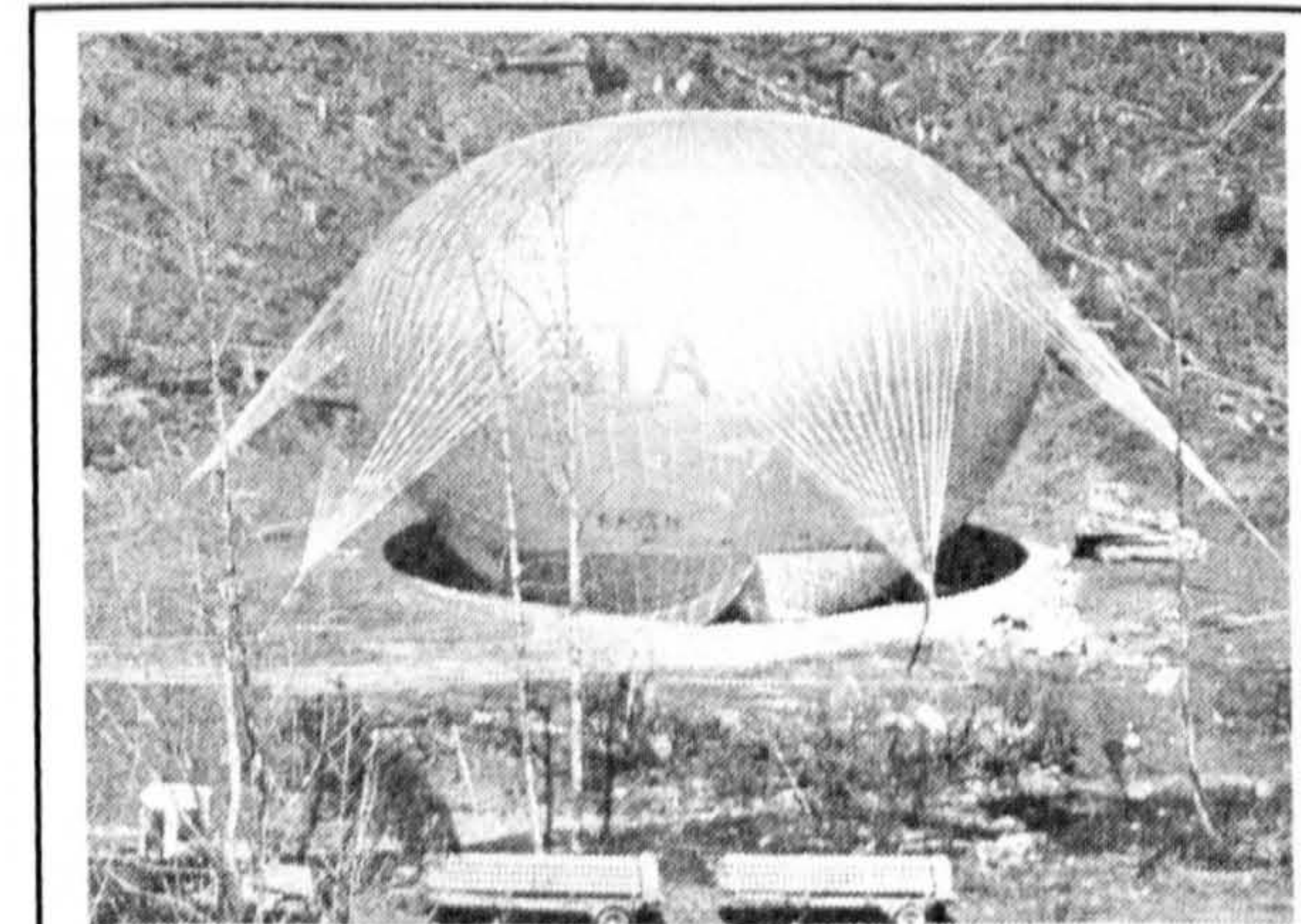
Figure 6.21 :1970 Canadian log-lifting balloon - note gas cylinders on trailers in foreground
